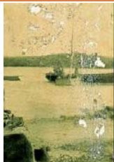
Cracking Emulsion on Photo
